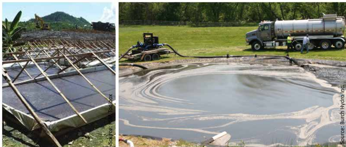
FIGURE 79: LIME STABILIZATION TECHNIQUES IN PHILLIPINES (LEFT) AND THE US (RIGHT)
