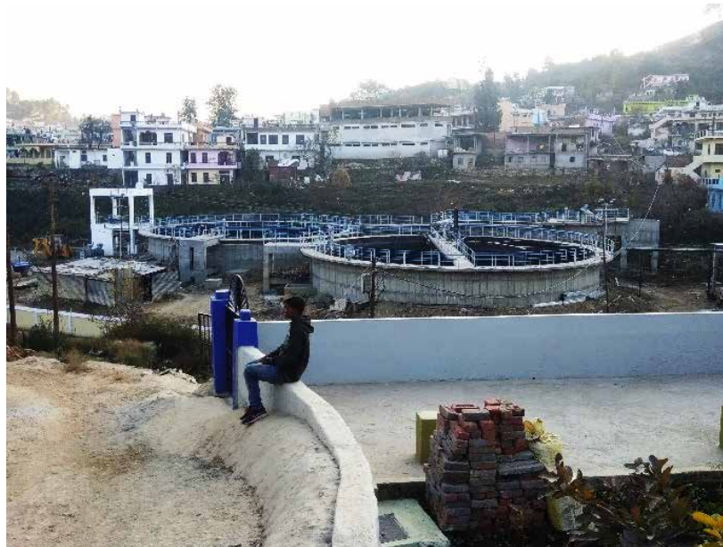
FIGURE 56: SEWAGE TREATMENT PLANT AT ANJOLI, PITHORAGARH OF 5 MLD CAPACITY
