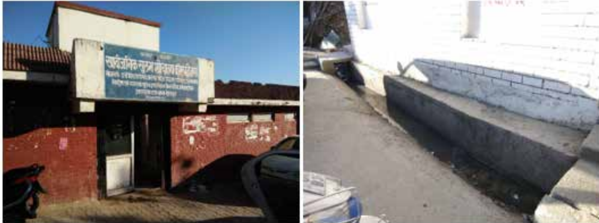
FIGURE 53: COMMUNITY TOILET WITH SEPTIC TANK AND OPEN DRAINS IN CITY AREA
