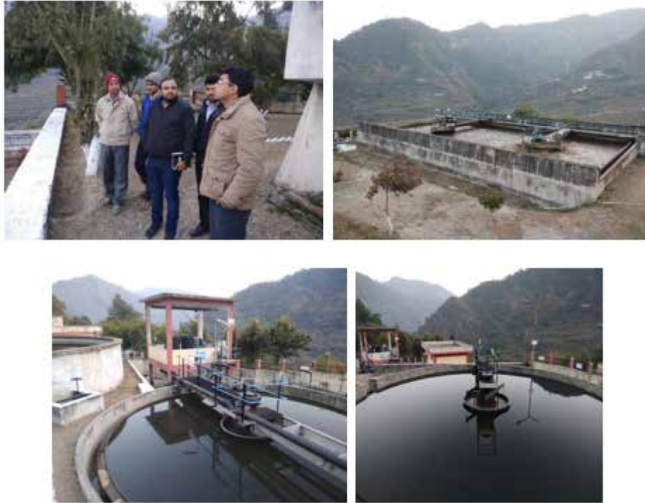
FIGURE 27: SEWAGE TREATMENT PLANT AT TEHRI WITH DESIGNED CAPACITY OF 5 MLD
